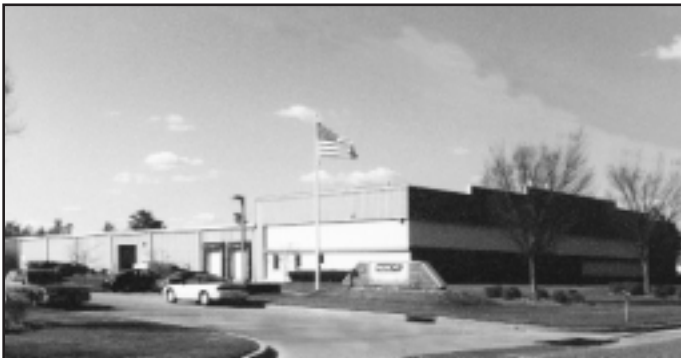
Manley Performance Products, Inc. Manufacturing Plant
